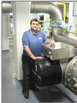
**The use of conventional treatment, chlorine disinfection, and UV disinfection are all part of the Water Filtration Plant multiple barrier treatment philosophy.** In this approach, different types of disinfection are used at different points in the treatment process to ensure the elimination of microorganisms found in Lake Michigan water. UV disinfection follows filtration and precedes chlorination.
